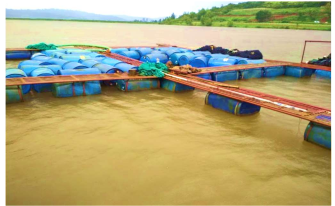
Fabrication of cages using locally available low cost materials in Andur reservoirs at Kolhapur
